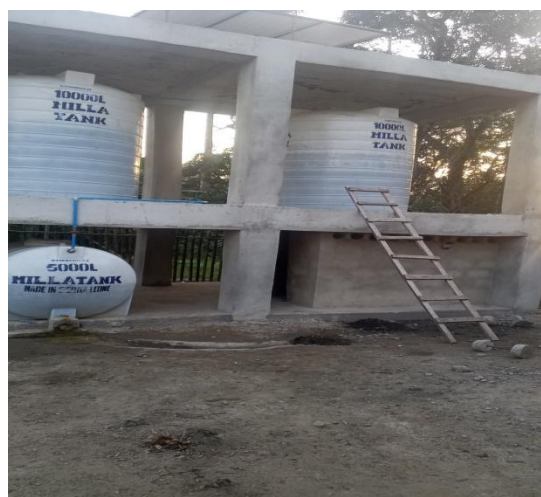
Misaligned Column Tower and Rough Dry floor slab (Mahera, Mambolo Chieftdom)
